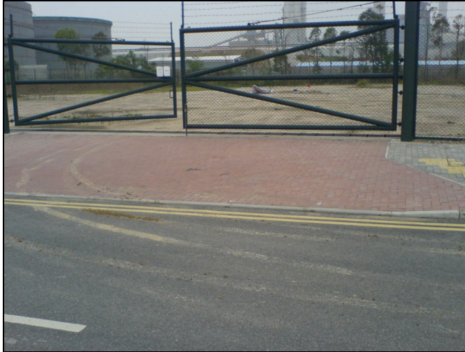
Photograph 8-1 Soil Debris on the Road Outside EP08-01
